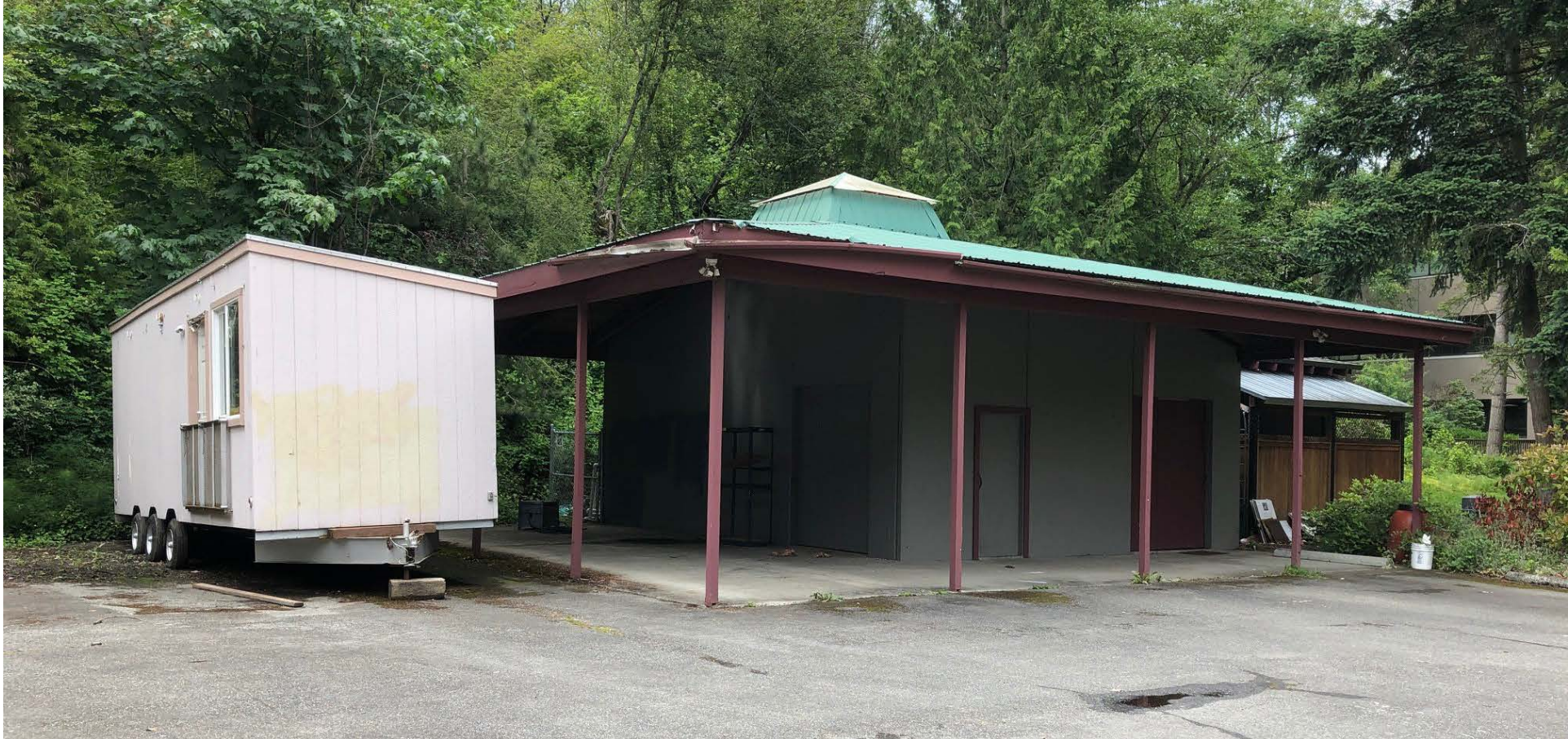
Recycling Center (looking northwest)
