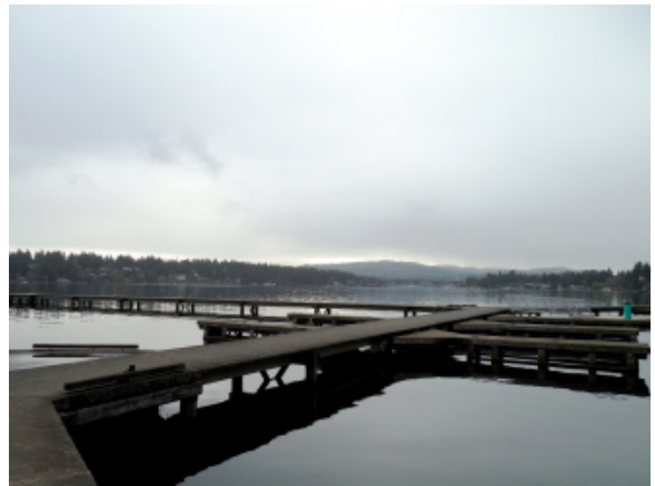
Photo 6A – Large pier
