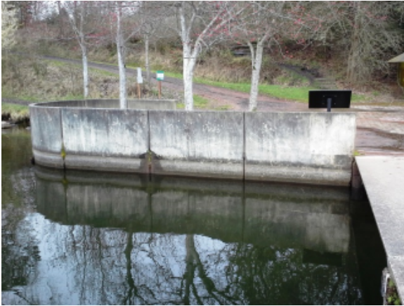
Photo 1A – Concrete bulkhead
