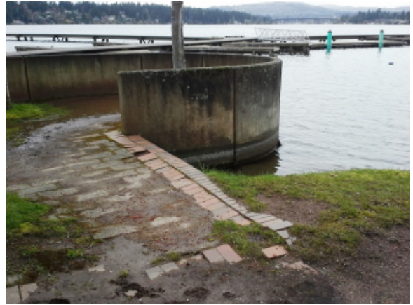
Photo 2A – Brickwork adjacent to bulkhead
