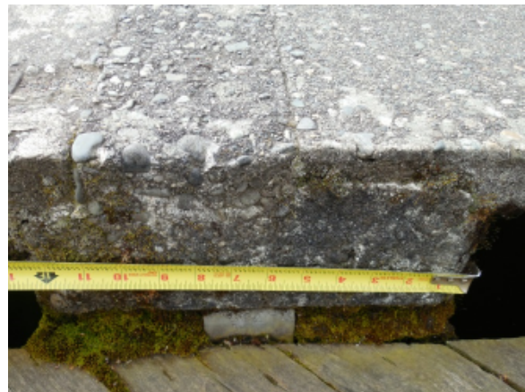
Photo 10A – Pier slab over support
